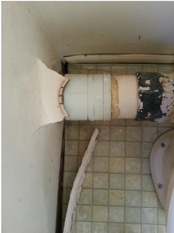
Figure 112. Pipe from WC & peeling skirting board (left) Figure 113. Bathroom south west corner (right) LK March 2014
