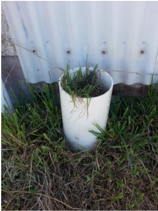
Figure 75. Old downpipe connection (left) Figure 76. Sheet connection detail (right),) LK March 2014
