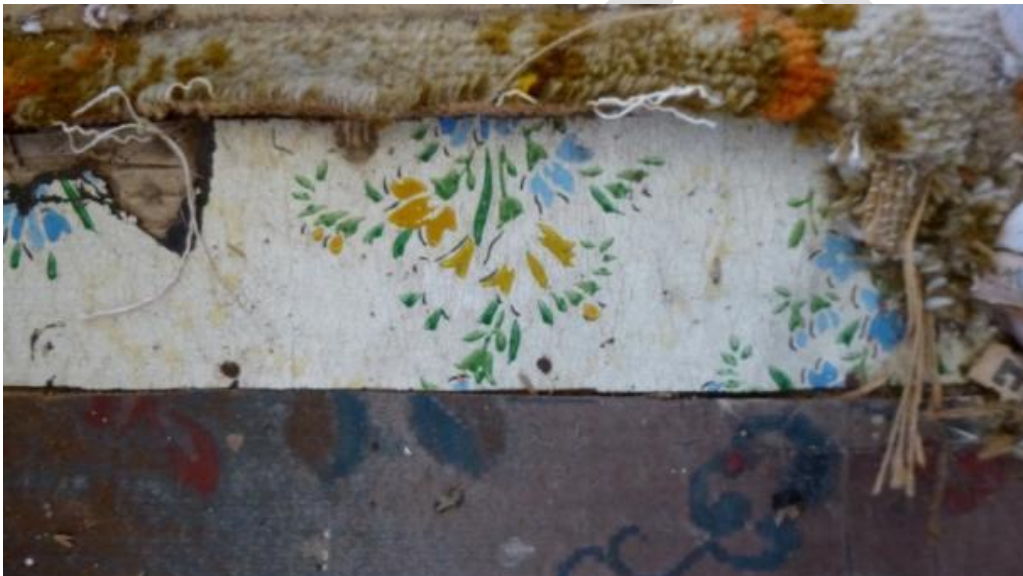
Figure 142. Layered flooring in bedroom, GB March 2014
