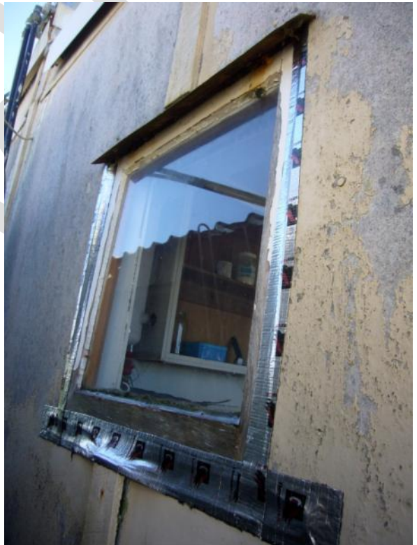
Figure 97. South wall, view west, showing pipes between crib and neighbouring shed (left) Figure 98. Kitchen window detail, showing temporary weathering repairs (right), GB March 2014
