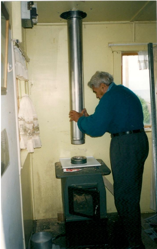
Figure 50. Hone fitting the flue, 2002. Photograph: Jeremy Hay
