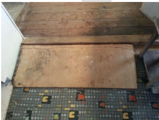
Figure 116. Linoleum patchwork on kitchen floor (left) Figure 117. Electrical socket detail below window on east wall (right) LK March 2014
