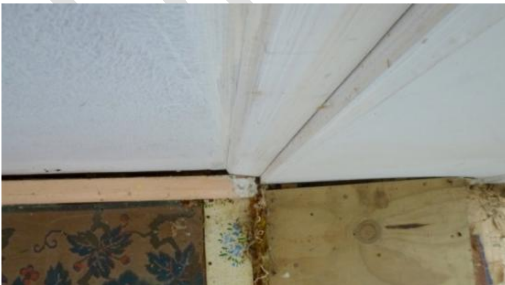
Figure 143. Ramped floor into bedroom at doorway, GB March 2014
