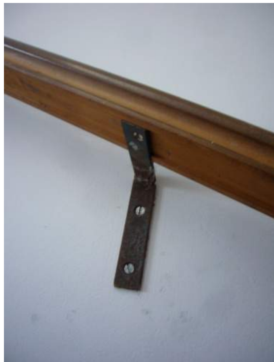
View west from staircase up into upstairs bedroom (left) Handrail detail – steel angle brackets (right)
