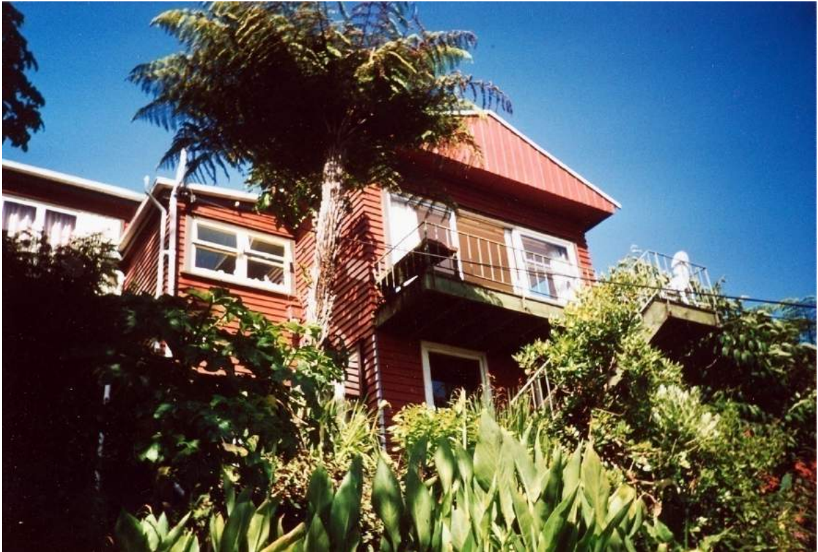
Shadbolt house, western façade 1996/7 Photo: Shadbolt family archives
