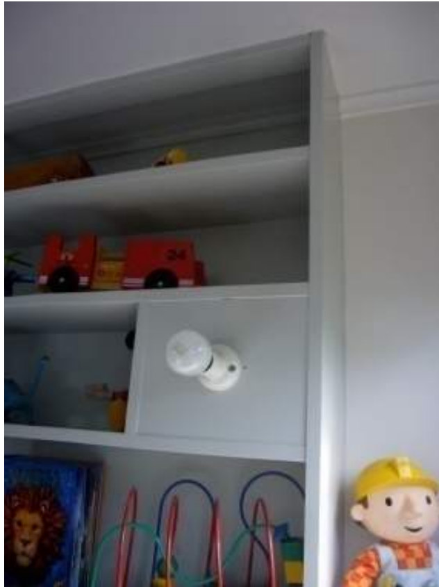
Exposed light bulb lamp wired into bookcase Photograph: Burgess & Treep 2013
