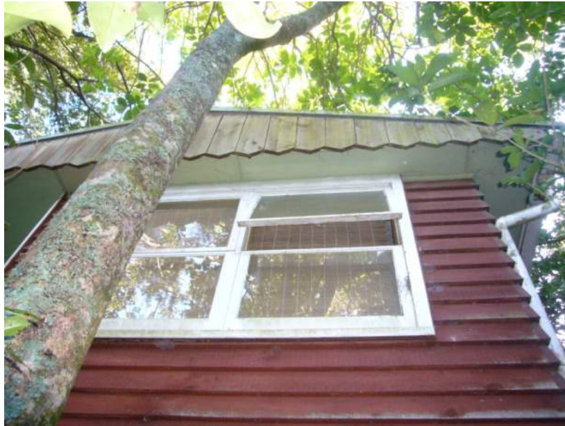
East wall of studio showing gable end detail and stacks of awning windows (Burgess & Treep 2013)
