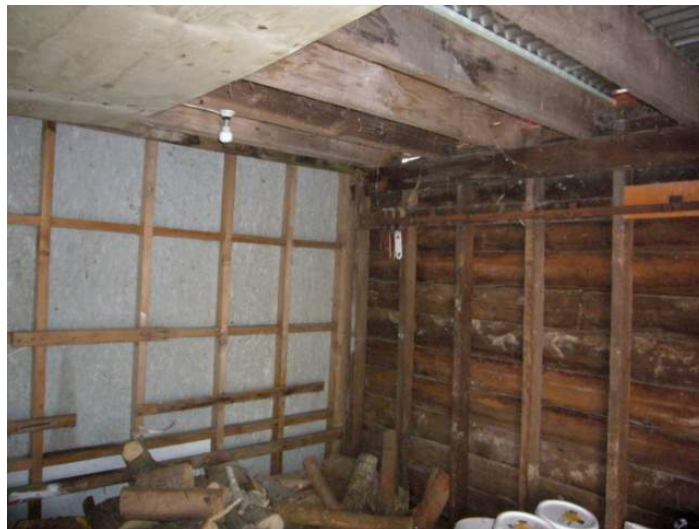
Interior of garage showing exposed framing (Burgess & Treep 2013)
