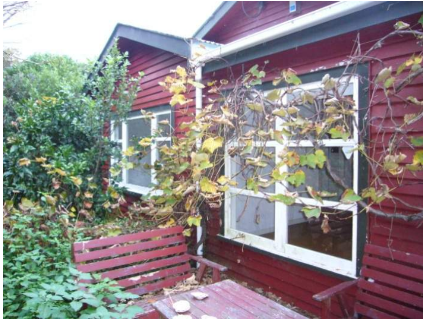
Eastern /street facade Photograph: Burgess & Treep 2006
