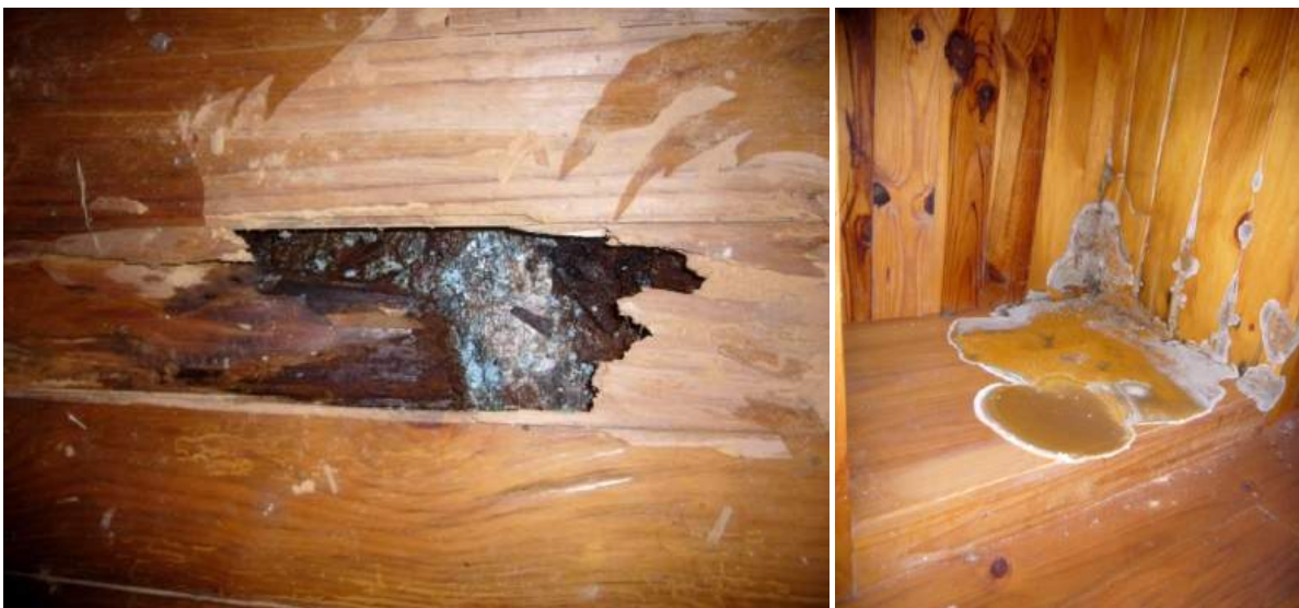
Rot in floor boards NB close proximity of timber to ground below (left) Mould in wardrobe (right) Burgess & Treep 2013
