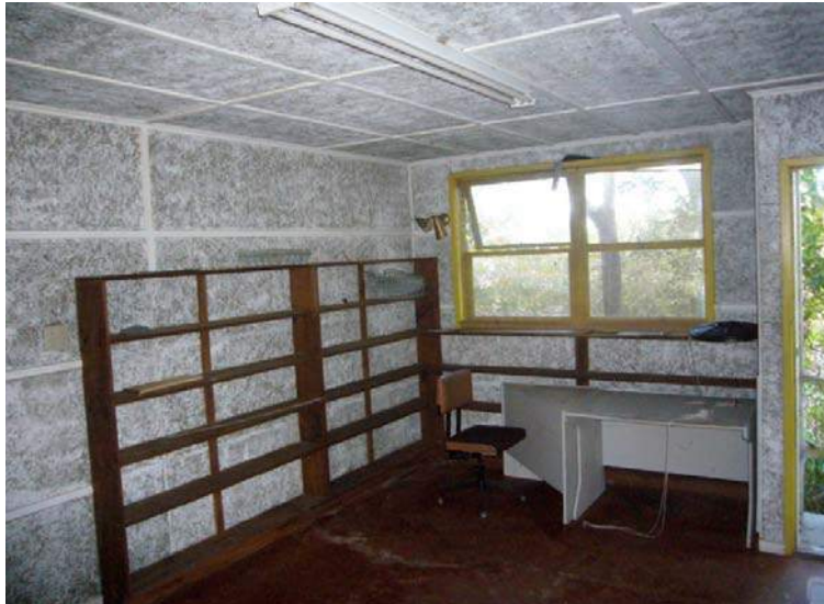
South wall of studio showing door to exterior (right) (Burgess & Treep 2013)
