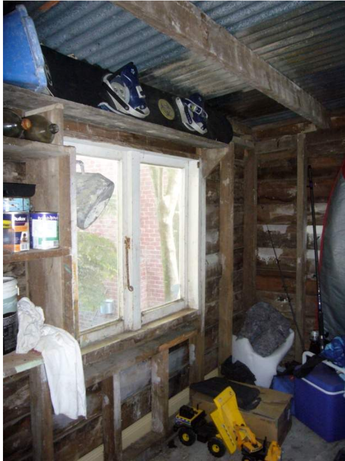
Interior of back room of garage (Burgess & Treep 2013)
