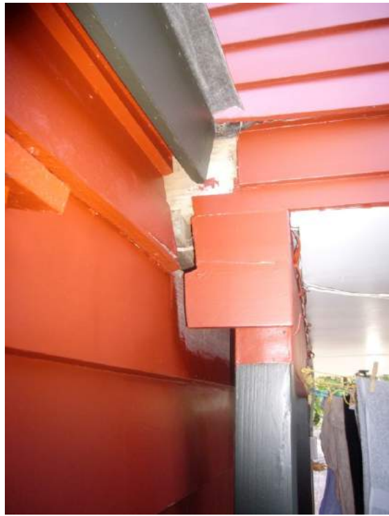
Photographs showing the significant movement of structural elements in garage (Burgess & Treep 2013)
