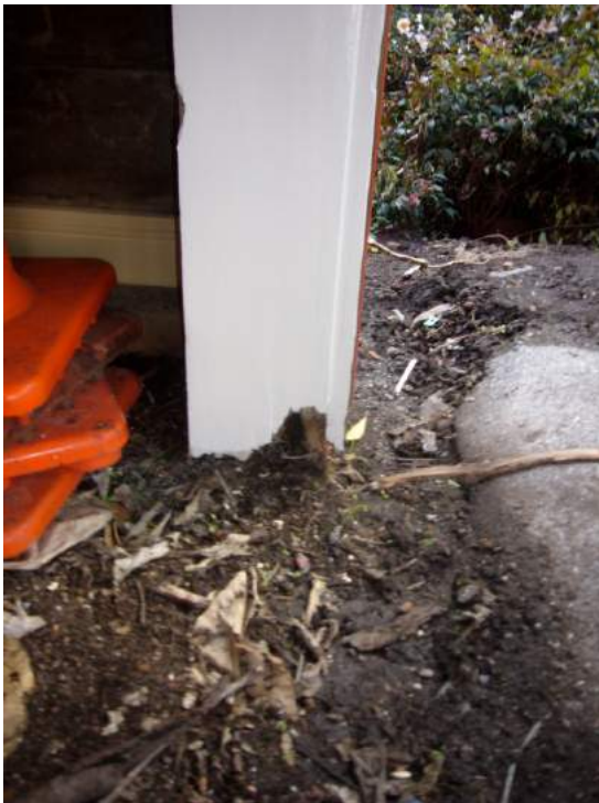
Movement of structure in garage (left) Timber built directly upon earth (right) (Burgess & Treep 2013)
