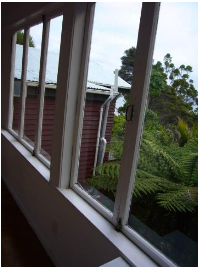
West wall showing rows of sliding folding windows with view out across bush to sea. Photograph: Burgess & Treep 2013
