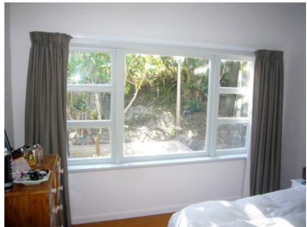
Built in cabinetry on west wall(left) picture window flanked either side by stacks of top hung awning window, east wall (right) Photograph: Burgess & Treep 2013
