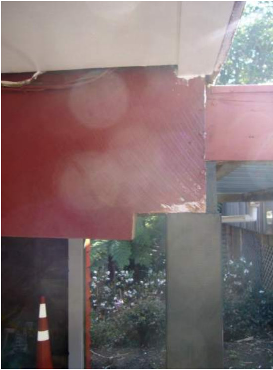
Photographs showing the significant movement of structural elements in garage (Burgess & Treep 2013)
