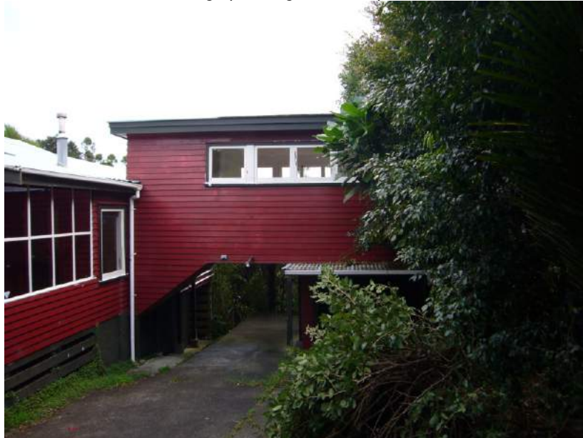
View west showing bedroom over garage Photograph: Burgess & Treep 2006
