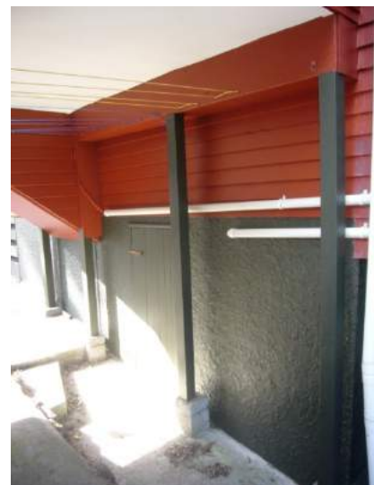
Garage beneath bedroom extension (left) Structure along supporting bedroom above garage (right) (Burgess & Treep 2013)
