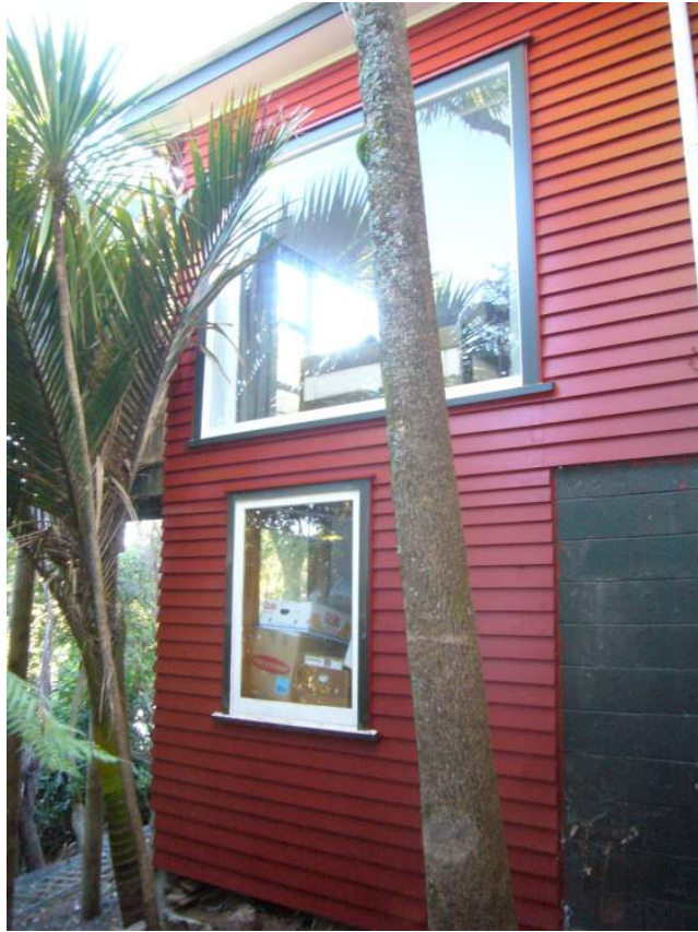
South wall of basement (Burgess& Treep 2013)
