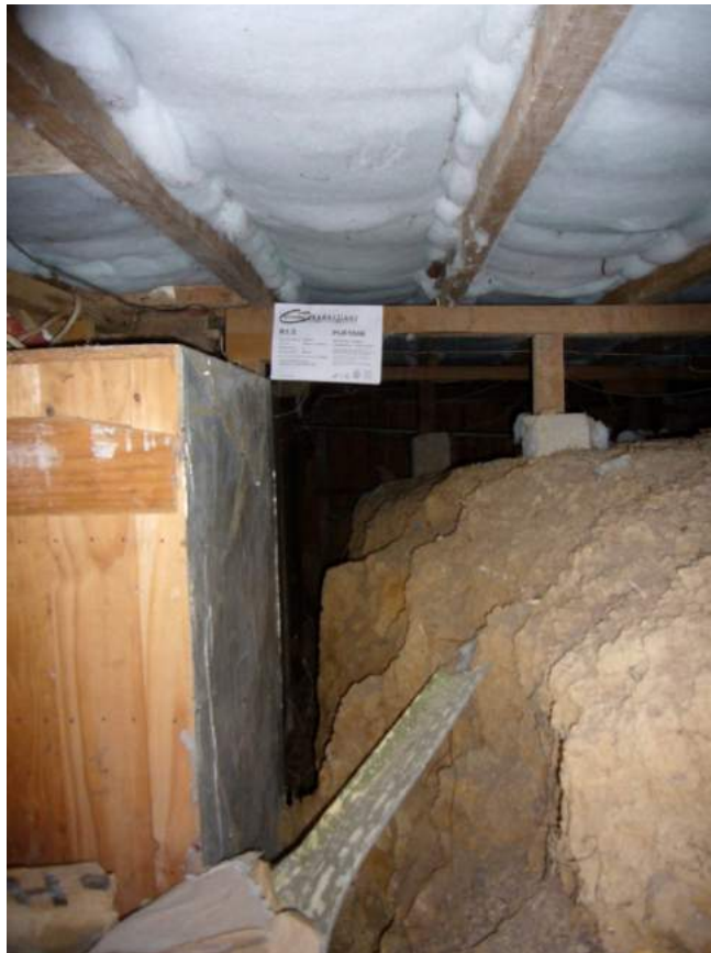
Exterior of basement showing block wall and unretained earth (Burgess& Treep 2013)
