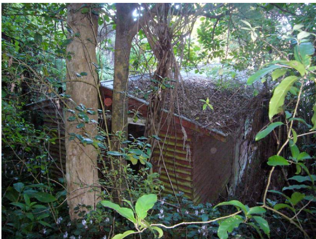
View down onto studio from path (Burgess & Treep 2013)
