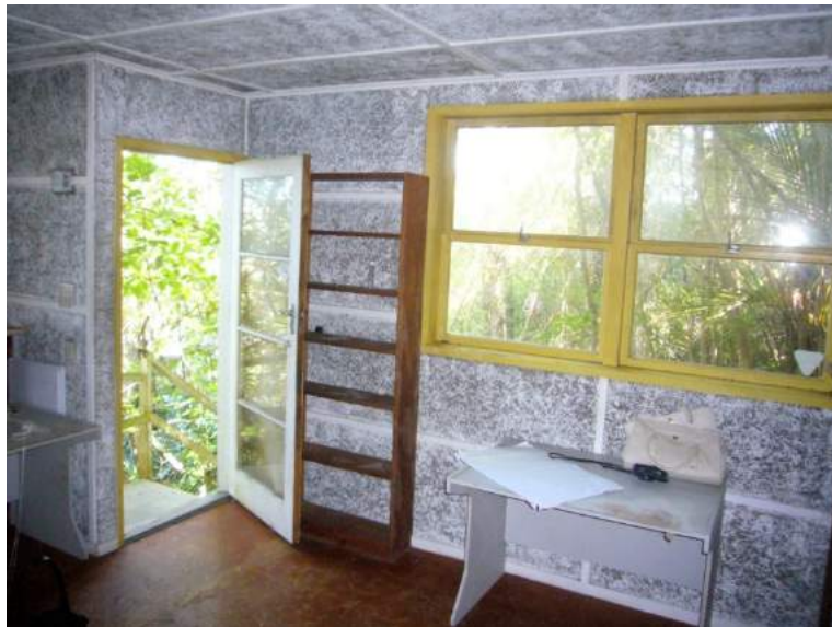
South-western corner of studio showing door to exterior (left) (Burgess & Treep 2013)
