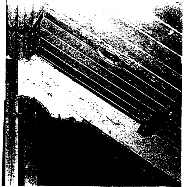
West Gable ceiling detail - truss Burgess & Treep, February 1996
