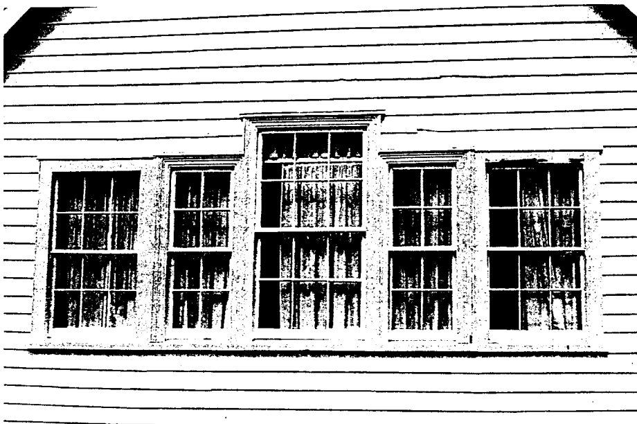
North Central Gable windows to classroom note rot to right hand window Burgess & Treep, February 1997
