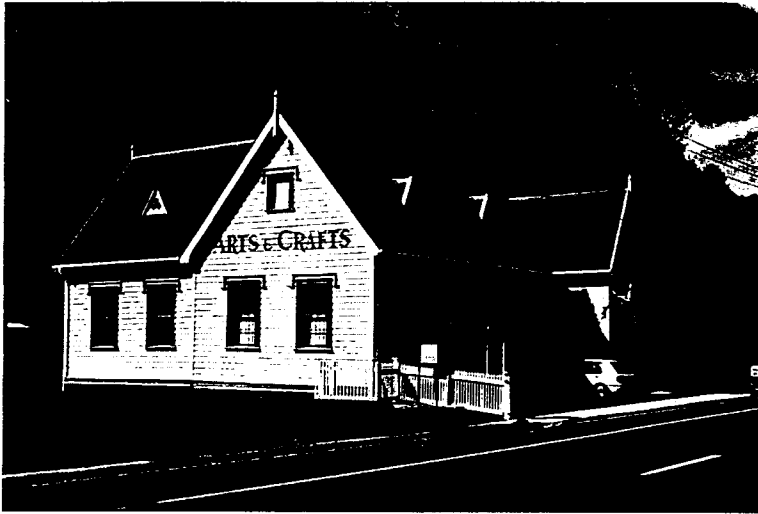
Thames North School, Photo Burgess & Treep
