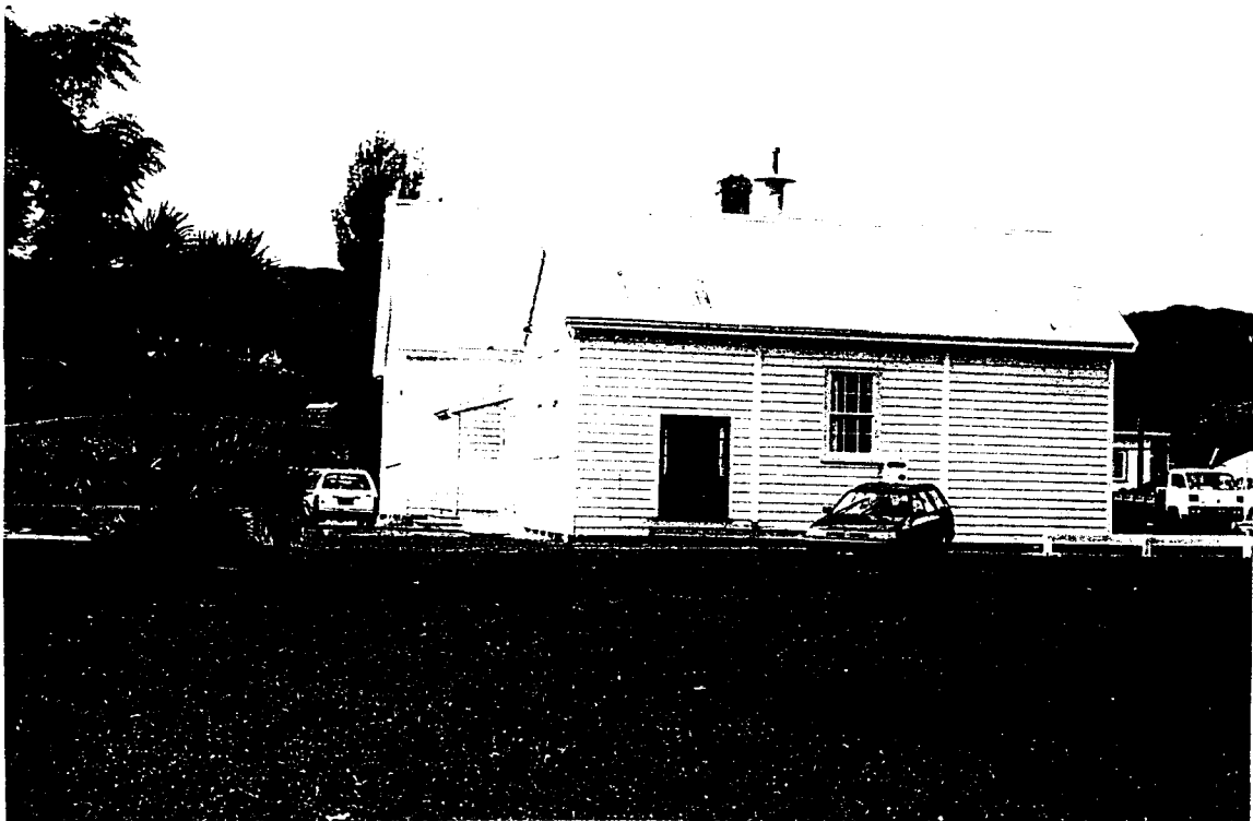
West Gable Burgess & Treep, February 1996
