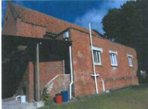
Figure 1.2: NW view of the church showing the Western annexe.
