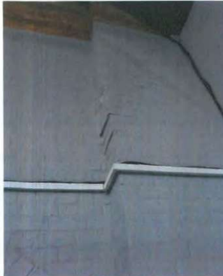
Figure 3.4: Masonry cracking and displacement in the Southern wall.
