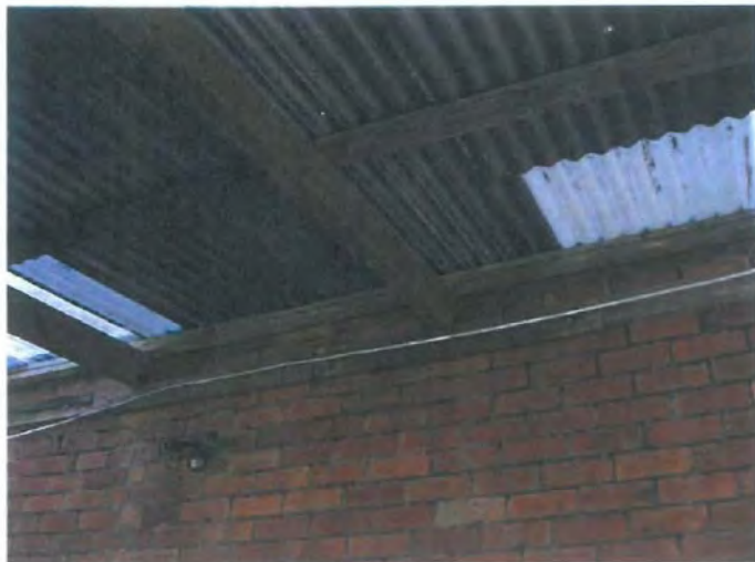
FIG 16: Shelter connection to North wall
