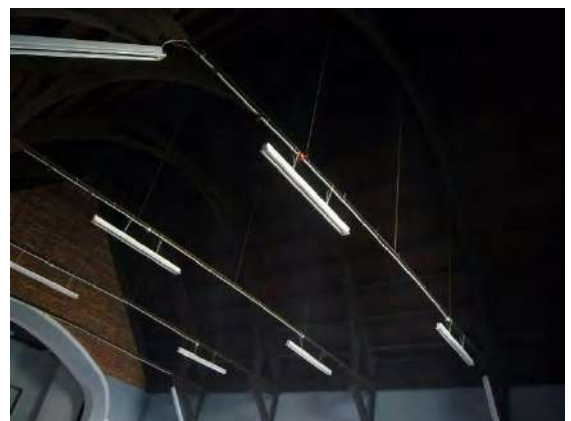
Looking up into the roof space showing the decorative timber trusses with steel tie rods and brick corbels. Note intrusive fluorescent light fittings hung from metal tie rods and mounted directly to trusses. Photograph: Lilli Knight, June 2016
