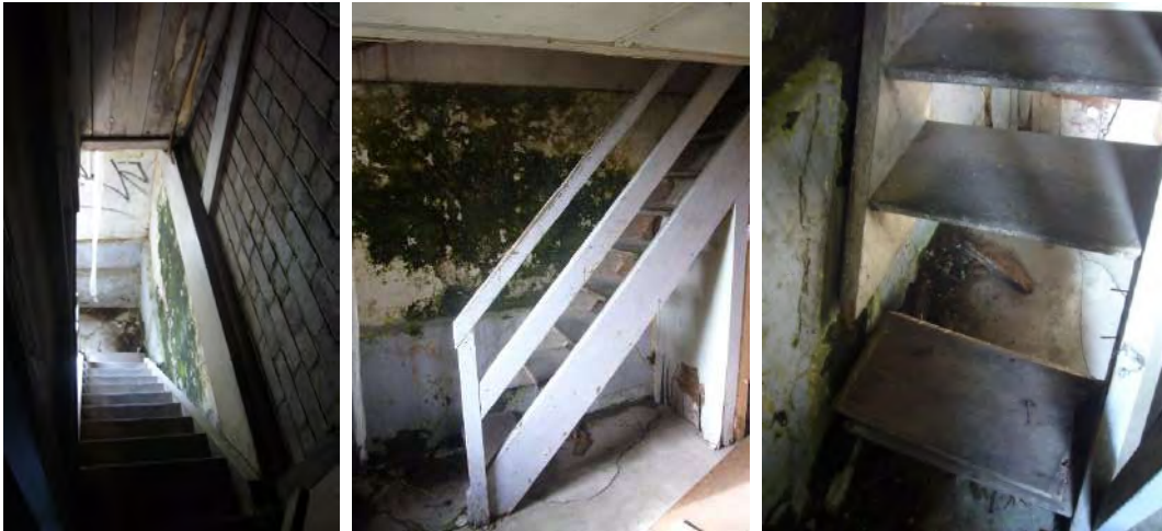
Showing timber stair with wooden treads, open risers down to basement from stage. Photographs Lilli Knight 2016
