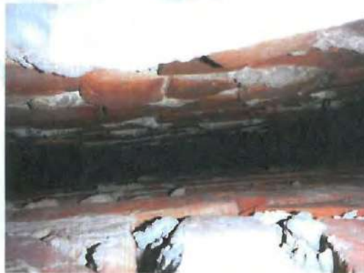
Figure 3.8: View of Eastern facade cavity showing failed masonry ties.
