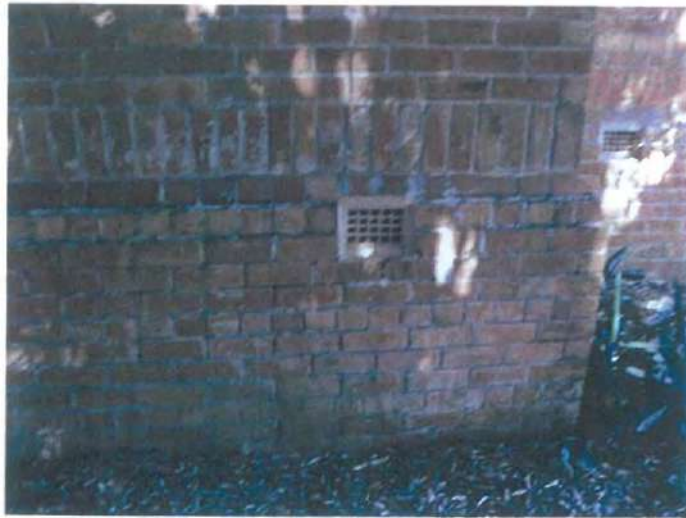
FIG 11: Mortar loss of outer skin
