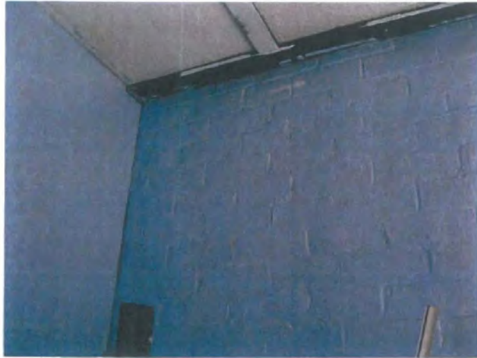
FIG 19: General internal cracking
