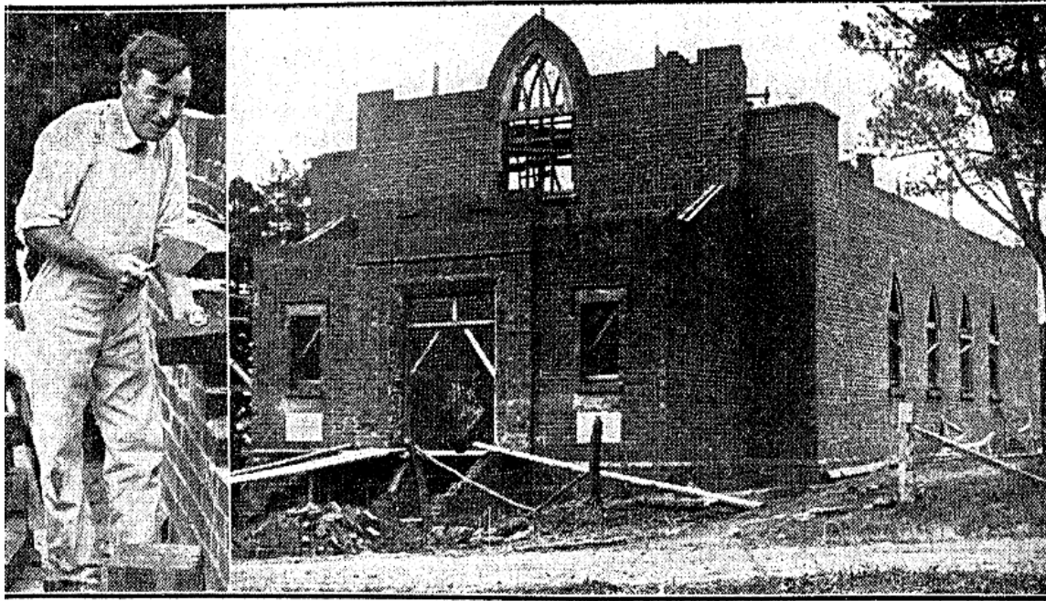
PROGRESS ON NEW SUNDAY SCHOOL FOR NEW LYNN PRESBYTERIANS. This building is being personally erected by the minister, the Rev. W. R. Rankin.
