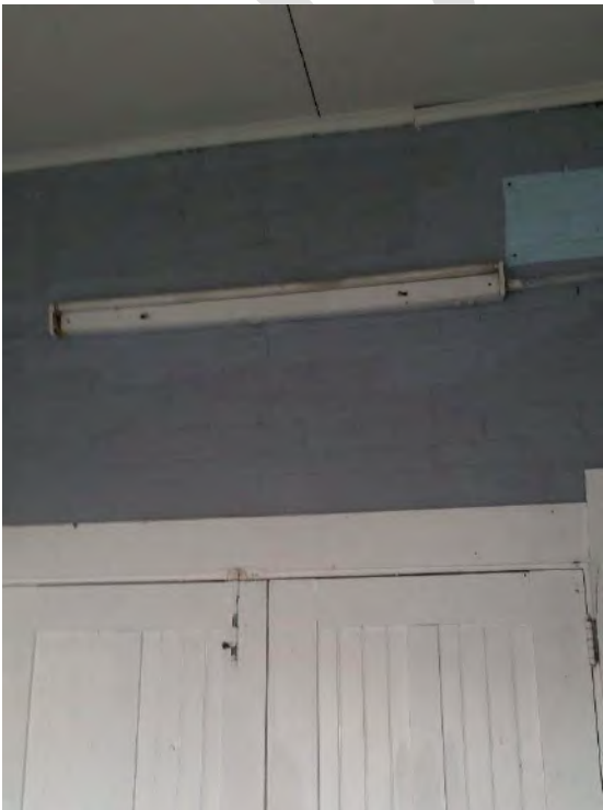
Showing north wall of entry vestibule. Fluorescent light fitting mounted on wall above double doors (left) historic distribution board and exposed wiring at north west corner of entry vestibule (right) Photograph: Lilli Knight 2016
