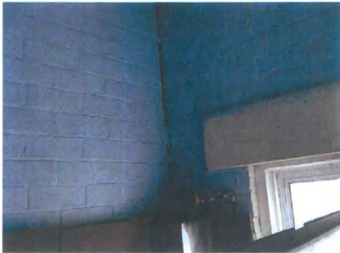
FIG 24: Disjointed internal wall
