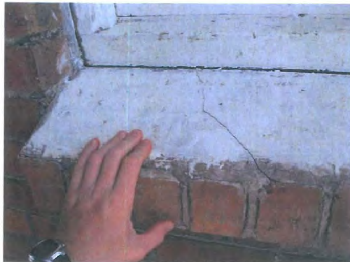
FIG 8: Sill cracking below arched window on East wall bulge
