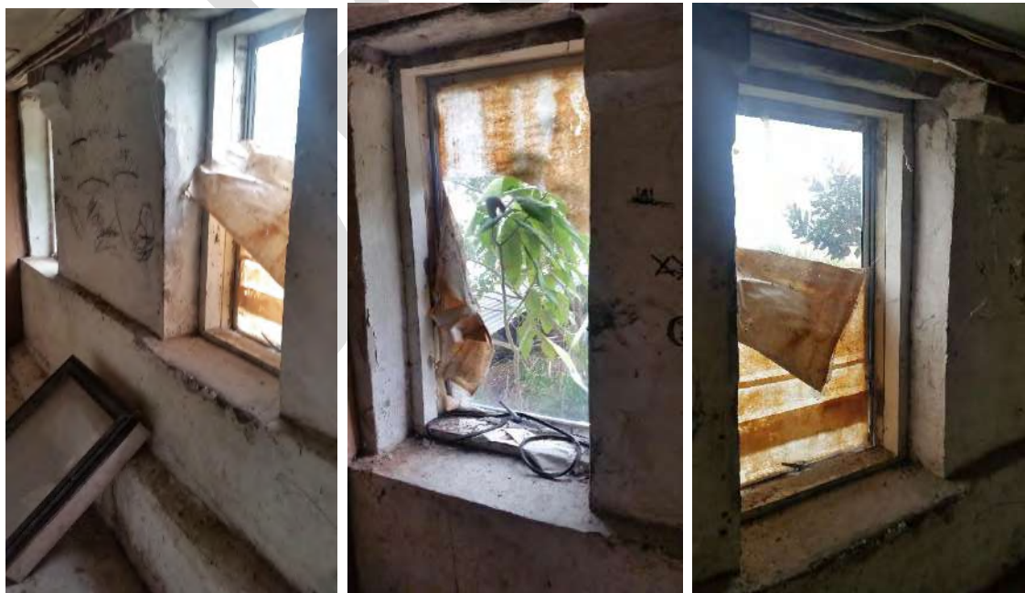
Showing windows added in the 1940s to the basement area. Original timber frame remains; timber sashes have been replaced with aluminium. Photographs: Lilli Knight 2016
