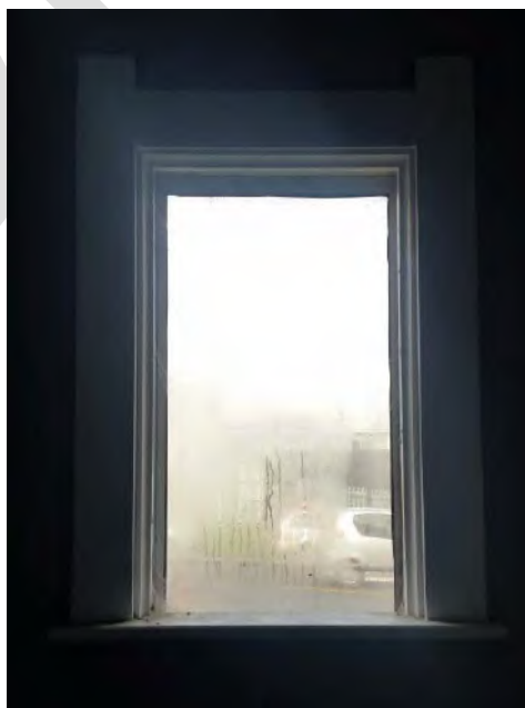
Left: Aluminum entry doors fitted into existing timber frame (left) aluminium window, fitted into existing timber frame with flat board timber architraves with projecting vertical detail (right) Photograph: Lilli Knight 2016
