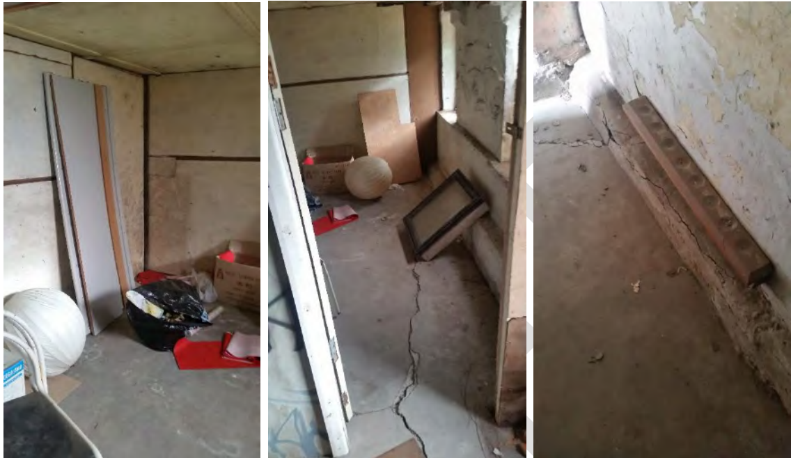
Showing partition walls in basement area (left) crack in plastered concrete floor (middle) pool cue holder fixed to south wall (right). Photographs Lilli Knight 2016
