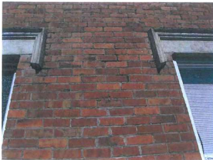
FIG 12: Mortar loss of outer skin
