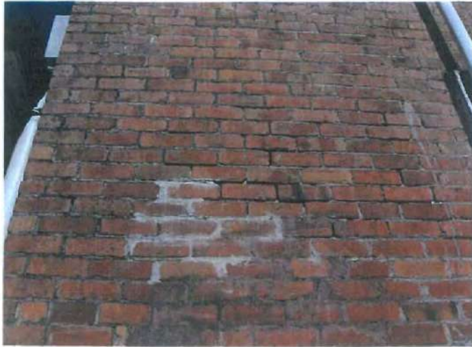
FIG 14: Mortar loss of outer skin
