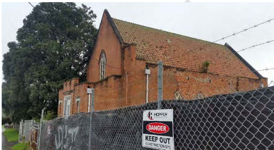
East elevation as viewed from Margan Avenue. Note brick collapse. Photograph: Lilli Knight 2016
