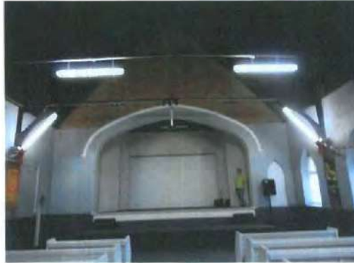
Figure 1.4: Interior of the church looking North at the stage.
