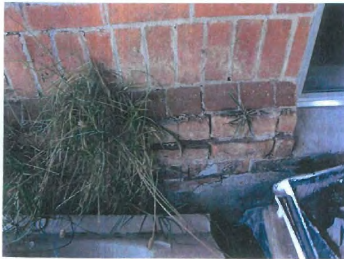
FIG 10: Mortar loss at foundation wall outer skin
