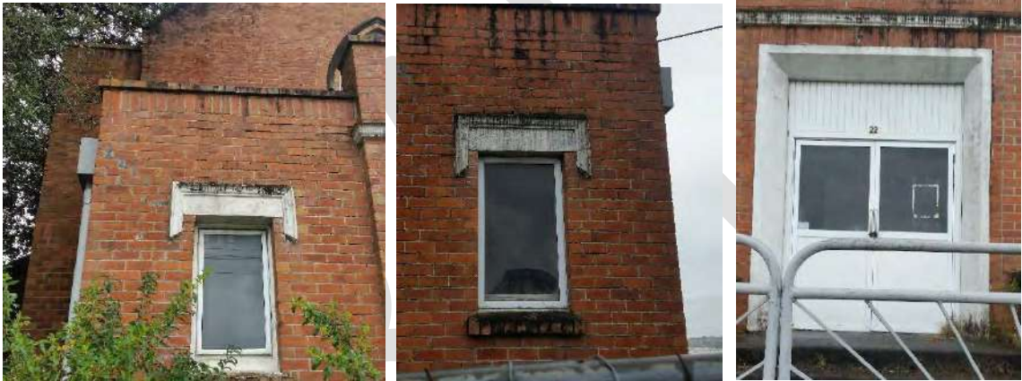
Windows on South façade (left) and original entry doors, replaced with aluminium joinery. Photographs: Lilli Knight 2016
