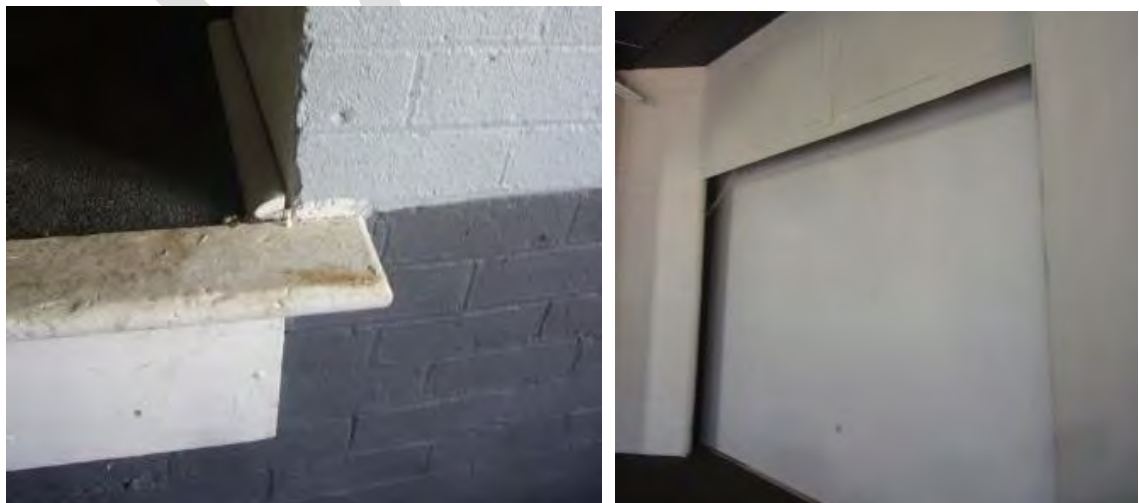
Plastered sill detail with flat faced sub board to proscenium arch (left) scenery backdrop at rear of stage (right) Photographs: Lilli Knight 2016
