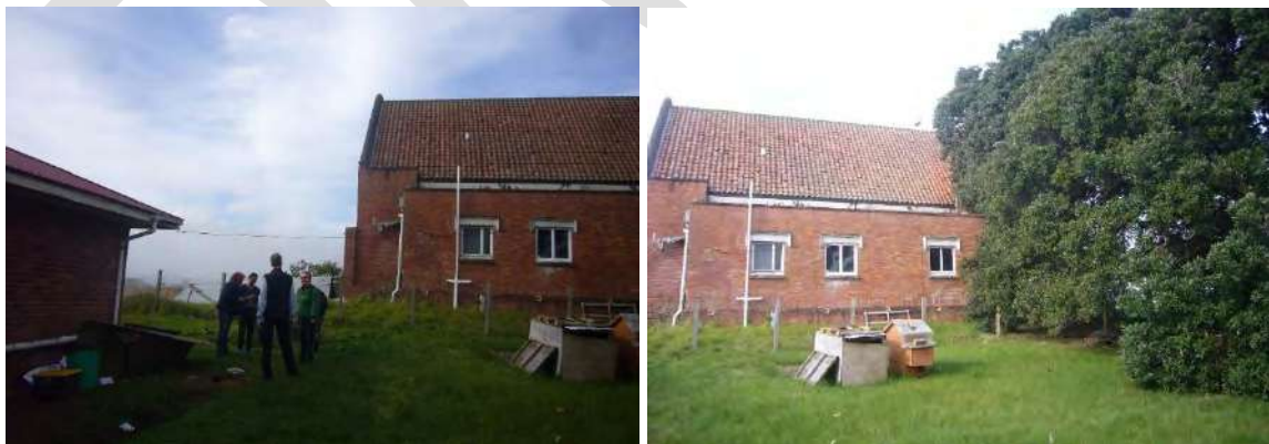
Showing west façade as viewed from Rankin Avenue. Photograph: Lilli Knight 2016
