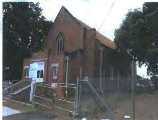
Figure 1.1: View of the South-Eastern Corner of the Church.
