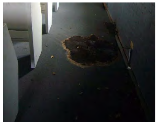
Showing brick movement on the east wall under windows (left) and on the south wall (middle) Water damage causing rot to floor boards along east side of the hall (right) Photograph: Lilli Knight, June 2016
