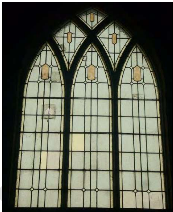
Showing one of the timber framed gothic arch windows set into east wall of the hall (left) large decorative lead light window with tracery set up high into the south wall of the hall (right) Photograph: Lilli Knight, June 2016
