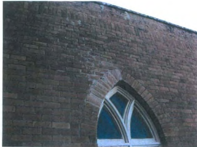
FIG 5: Patched repair above arched window on East wall bulge
