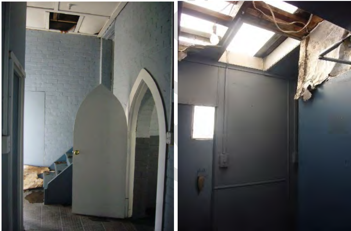
View through rear lobby towards female toilets, showing door way covered over, original doorway through to hall space on left and timber stair to stage behind (left) showing dilapidated state of female toilet addition (right) Photographs: Lilli Knight 2016
