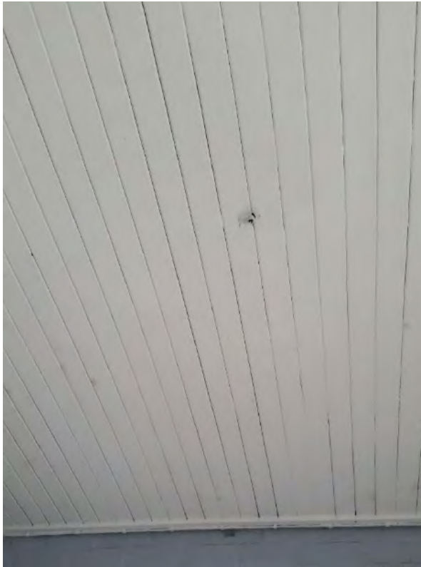
Match lining to ceiling in east ancillary room, remnant metal conduit at centre (left) decorative plaster ceiling panel in entry vestibule (right). Photograph: Lilli Knight 2016
