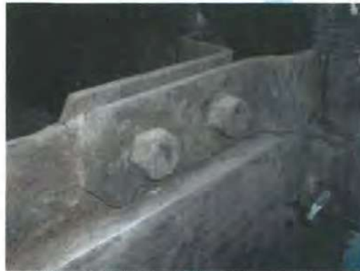
Figure 3.12: Arch tension tie to timber connection.
