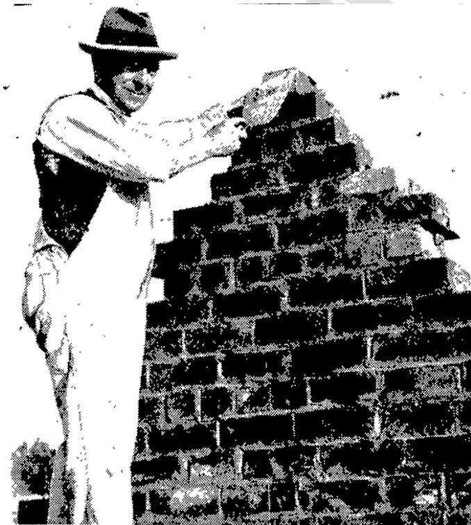
An Ambition Realised - The Rev. W. P. Rankin laying the last brick in the New Lynn Presbyterian Sunday School yesterday. Source: Auckland Star, Volume LX, Issue 121, 24 May 1929
