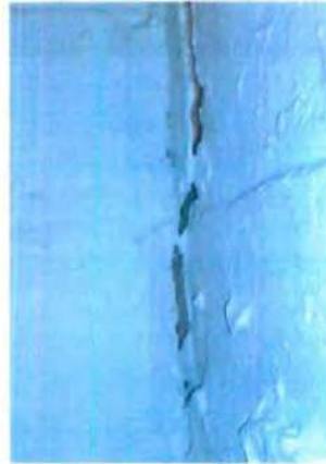
Figure 3.7: Cracking/Gapping at wall interfaces.
