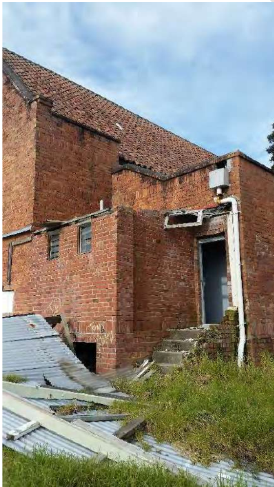
Showing the 1972 toilet addition at the north west corner (left) and the collapsed lean to at the rear of the building (right). Photograph: Lilli Knight 2016
