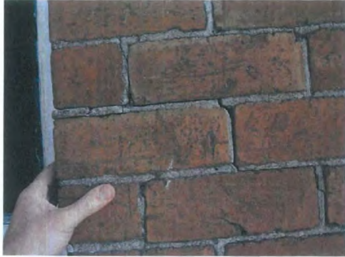
FIG 9: Loose outer skin brickwork beside arched window on East wall bulge
