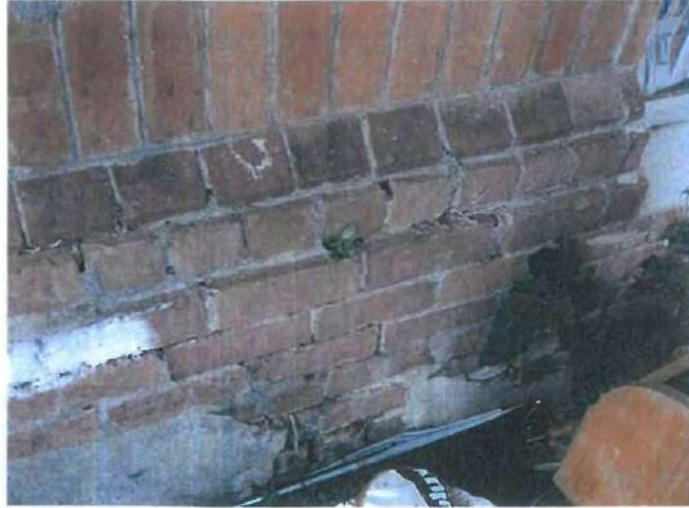
FIG 13: Mortar loss of foundation wall outer skin
