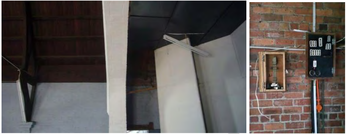
view up to the arch showing stage ceiling, underside of the brick proscenium arch and roof of the hall (middle) Old distribution board, stage (right) Photograph: lilli Knight 2016
