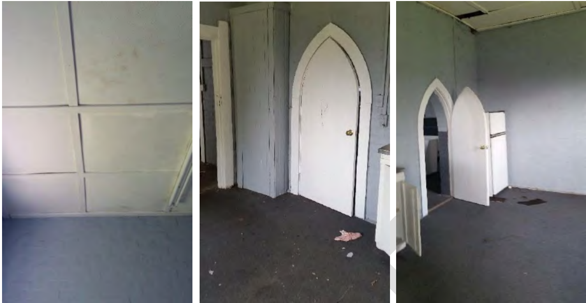
Showing plaster ceiling panels with timber battens (left) Gothic door through to hall, original t g v built in cupboard to left of door (middle) Showing gothic door leading into main hall at south end of the room (right) Photograph Lilli Knight 2016
