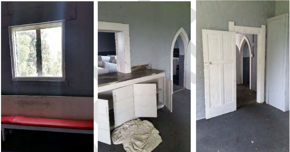
Showing aluminum windows sashes fitting into existing timber frames along west wall. Timber architraves remain (left) view of servery cabinetry, with stainless steel bech top (middle) showing timber framed t g v panel door with 'cross detail' in north end of the room leading into rear lobby. (right)
