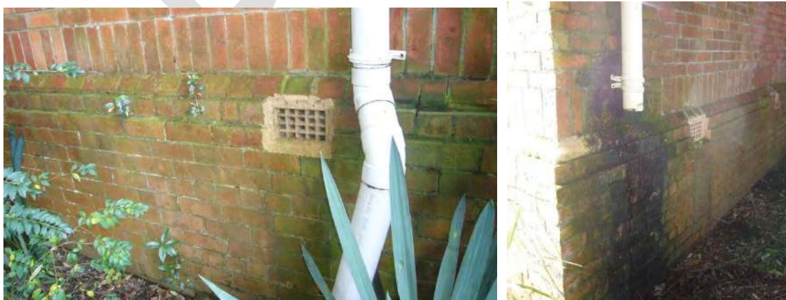
Showing brick vent set into foundation wall (left) down pipe disconnected, discharging onto brickwork (right) Photograph: Lilli Knight 2016
