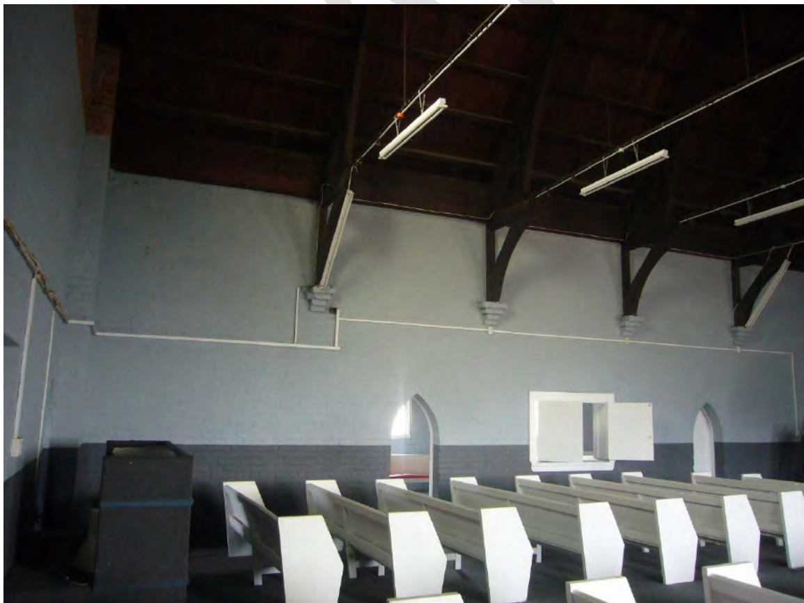
Showing the west wall of the hall, with doors into the classroom area + servery. Note wiring surface fixed in plastic conduit along wall. Photograph: Lilli Knight 2016
