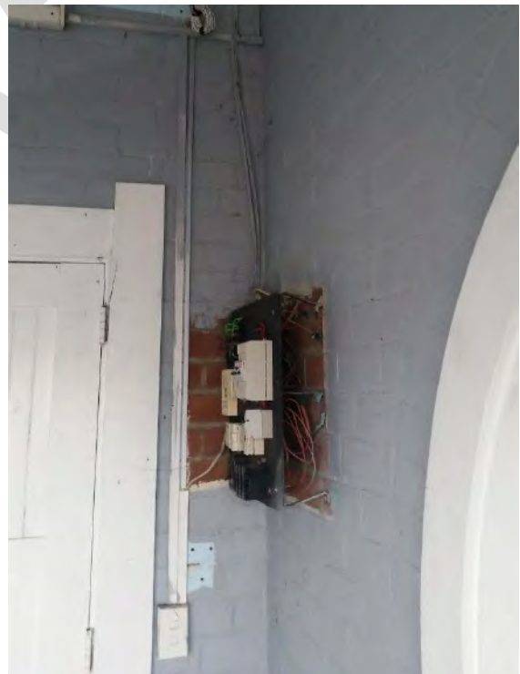
Showing north wall of entry vestibule. Fluorescent light fitting mounted on wall above double doors (left) historic distribution board and exposed wiring at north west corner of entry vestibule (right) Photograph: Lilli Knight 2016
