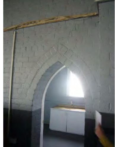
Showing window sill and architrave detail in east ancillary room (left) timber flat board architrave around gothic doorways (middle) view from hall looking through doorway into east ancillary room showing pointed arch brick detail around door way (right) Photograph: Lilli Knight 2016
