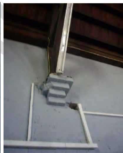
Commemorative stone set into east wall of the hall. Acknowledging the work of Reverend Rankin (left) brick corbel supporting truss, note hole cut into brickwork to allow for retrofitted electrical wires (right). Photograph: Lilli Knight 2016
