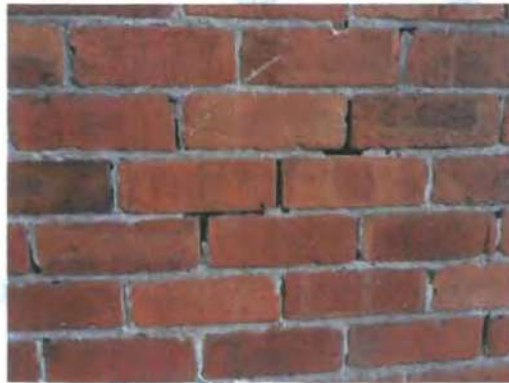
Figure 3.1 Example of poor grouting and pointing around masonry.
