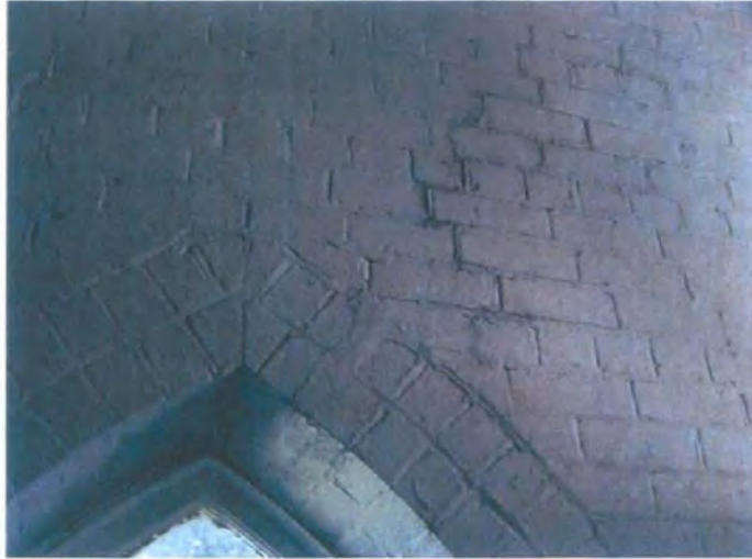
FIG 23: Internal cracking above arched window at outer skin bulge location on East
