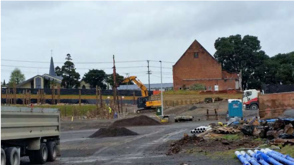
Showing the rear (north) face of the hall as viewed from the former brickworks site. Photograph: Lilli Knight 2016
