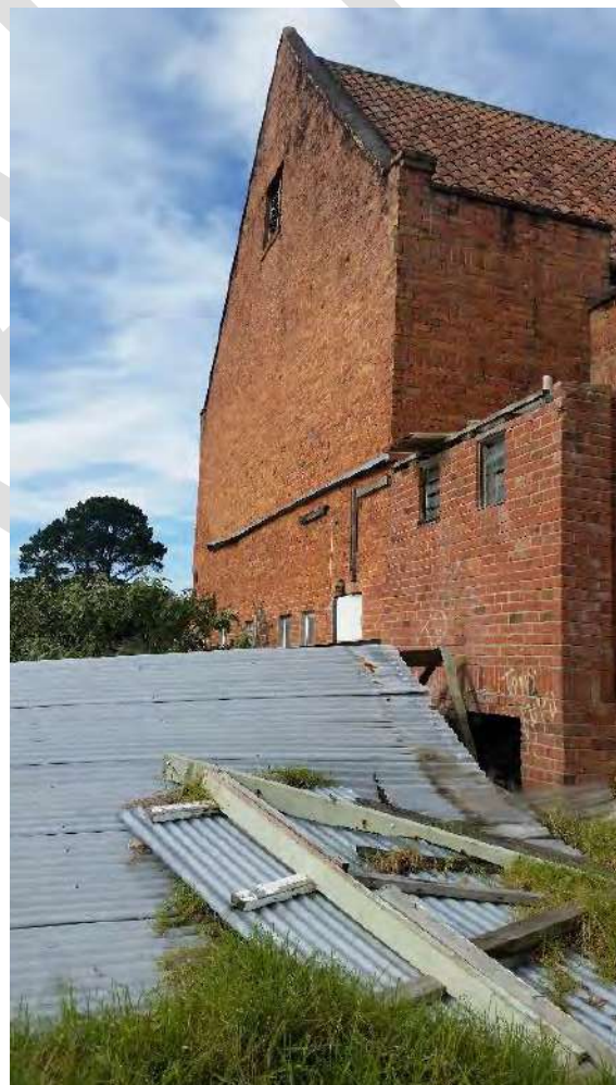
Showing the 1972 toilet addition at the north west corner (left) and the collapsed lean to at the rear of the building (right). Photograph: Lilli Knight 2016
