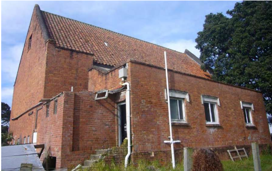
Showing north + west facades.
