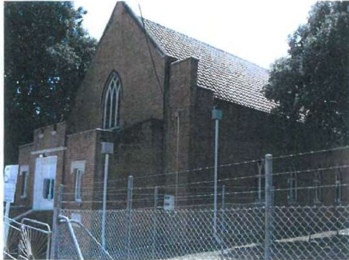
FIG 1: South wall, facing Margan Ave
