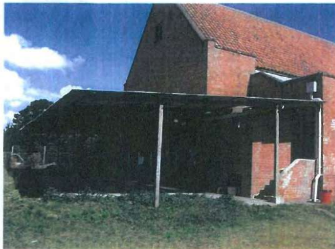
FIG 2: North wall & shelter
