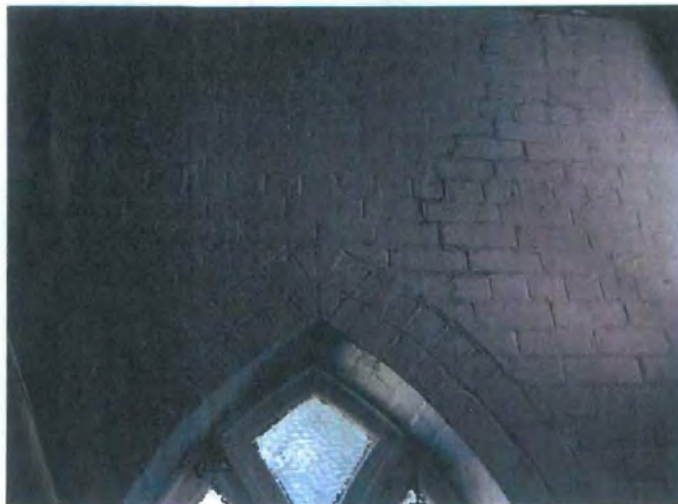
FIG 22: Internal cracking above arched window at outer skin bulge location on East wall
