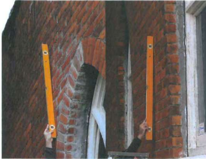
Figure 3.5: Curvature (bowing) in Eastern facade and cracking around windows.
