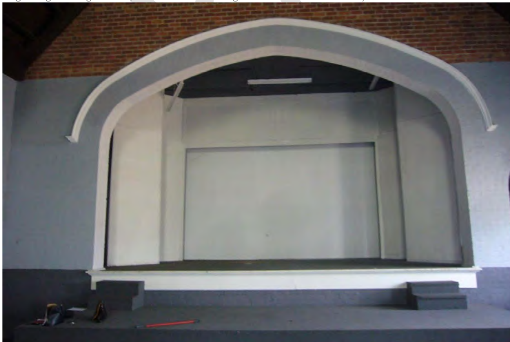
Showing the proscenium arch with plastered hood moulding and stage. Lower level stage is a later addition. Photograph: Lilli Knight 2016.
