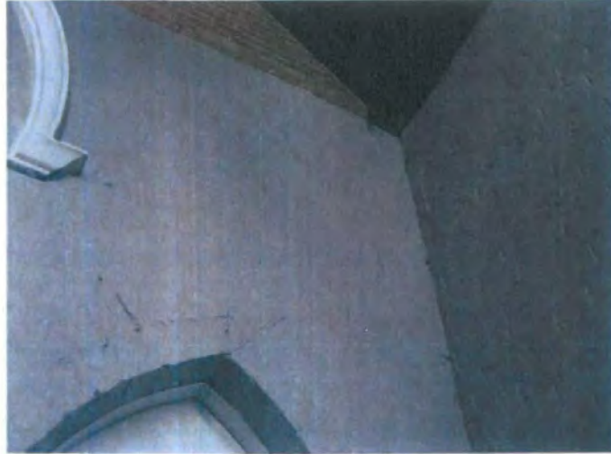
FIG 21: General internal cracking
