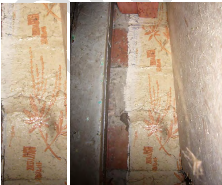
Showing stencilled paintwork remnant on brick walls. Photographs: Lilli Knight 2016
