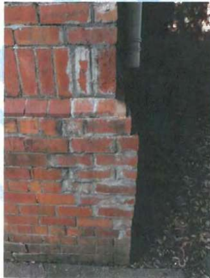
Figure 3.3: Poor repair work to cracking in masonry
