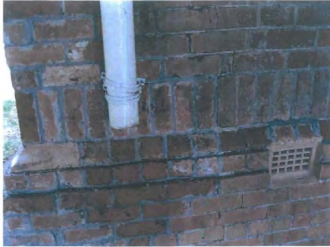
FIG 15: Disjointed downpipe
