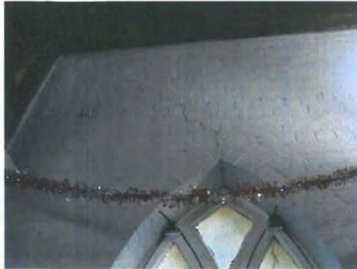
Figure 3.2: Cracking around windows in Eastern facade.
