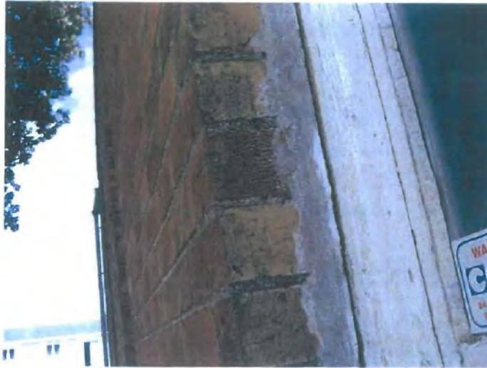
FIG 7: Previous repair around arched window on East wall bulge
