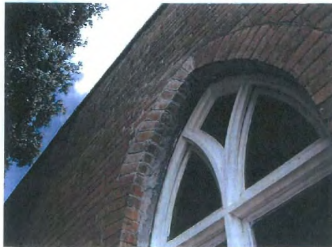
FIG 6: Cracking around arched window on East wall bulge
