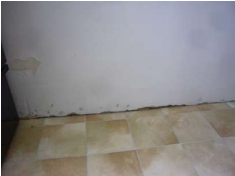
Base of west wall, Image: B&T Architects 2014
