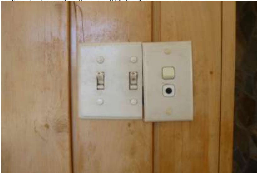
Switches at east end of hall, Images: B&T Architects 2014
