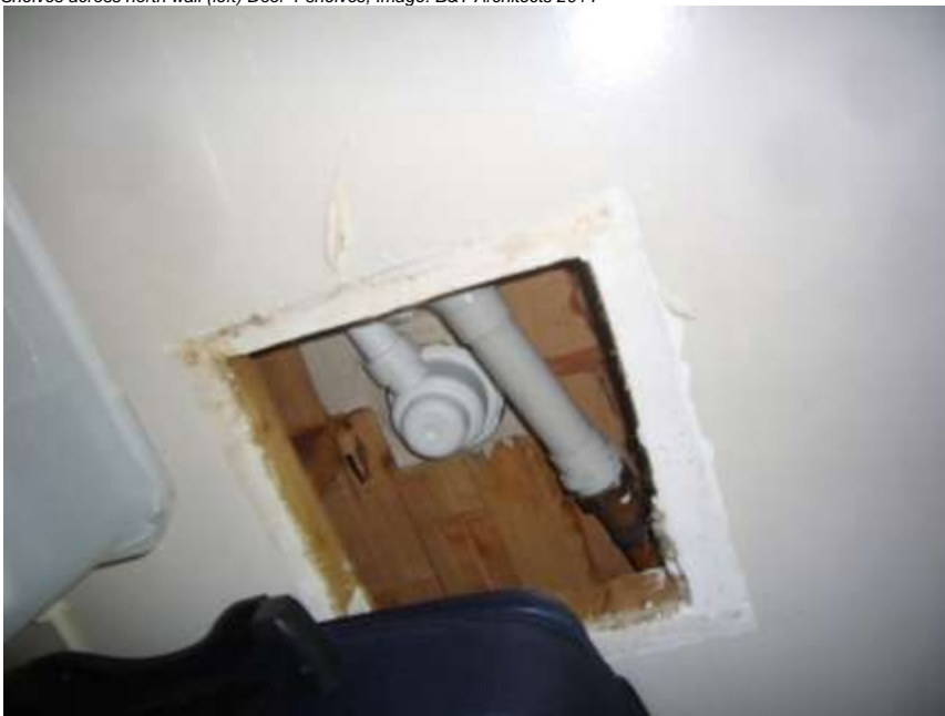
Plumbing access in ceiling, Image: B&T Architects 2014
