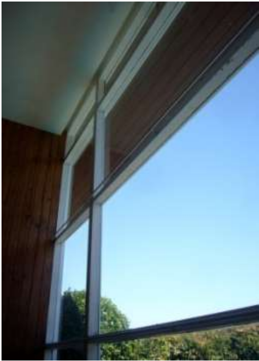
Double height joinery unit with structural steel rods (left) View across garden room from top of stair (right) Images: B&T 2014
