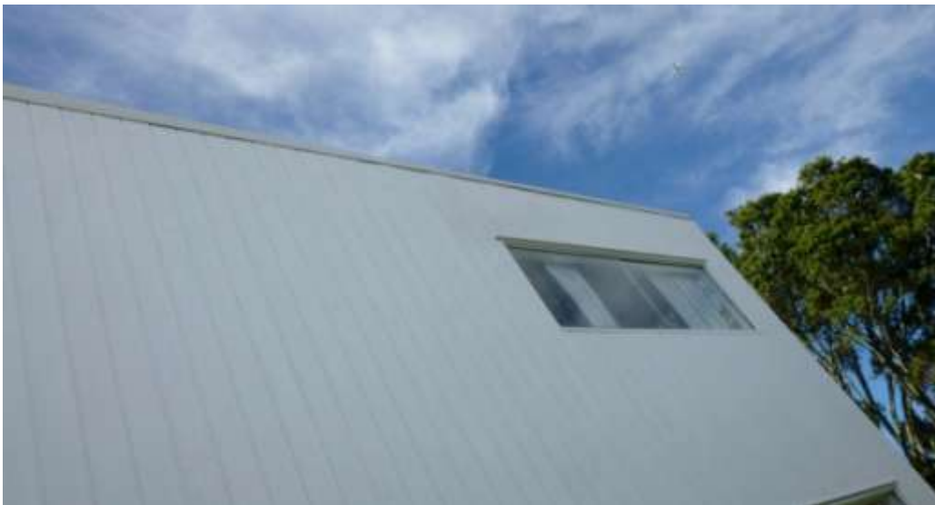
West Elevation, Image: B&T Architects 2014
