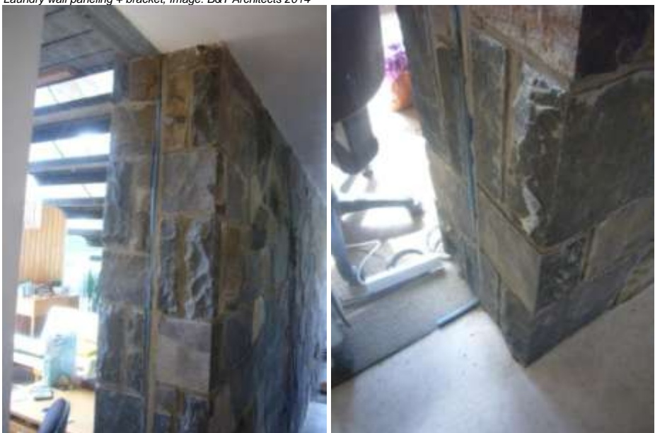
Stone wall + glass partition junction, top (left) Stone wall junction, bottom (right) Image: B&T 2014
