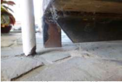
Post rust + stair prop (left) Step prop (right) Images: B&T Architects 2014
