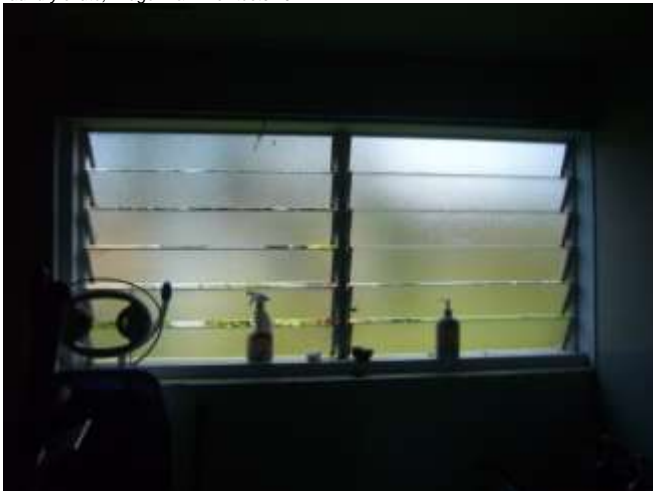
Louvered windows along south wall, Image: B&T Architects 2014
