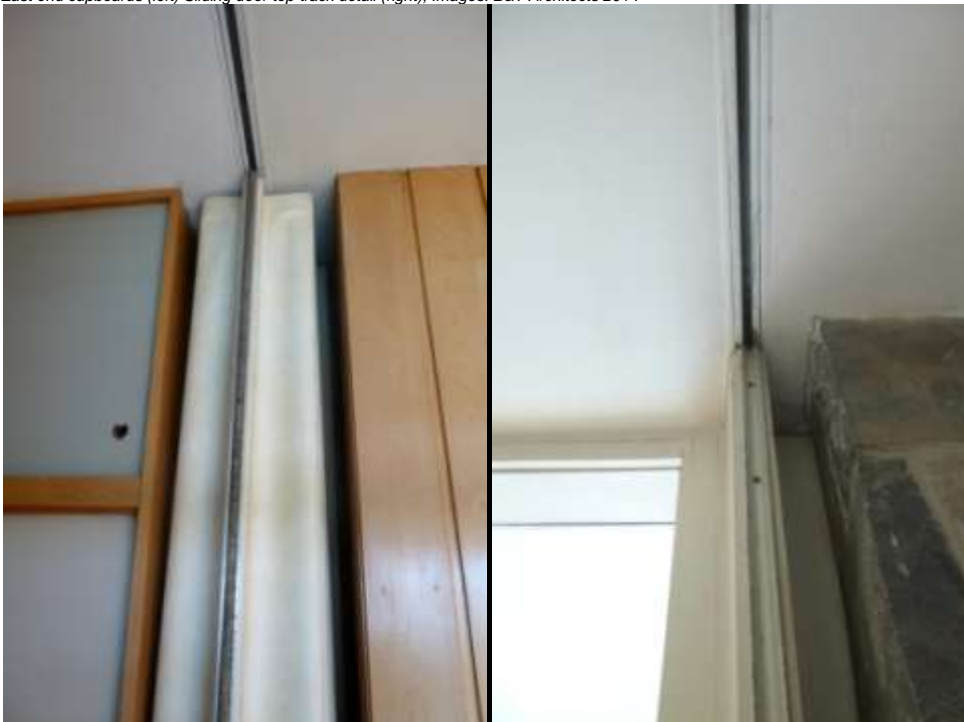
Concertina door open position south wall (left) Sliding door top track detail (right), Images: B&T Architects 2014
