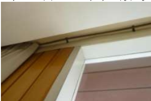
Recessed curtain tracks (left) Curtain track reveal detail (right) Image: B&T Architects 2014
