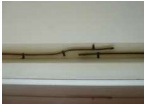
Recessed curtain tracks (left) Curtain track reveal detail (right) Image: B&T Architects 2014
