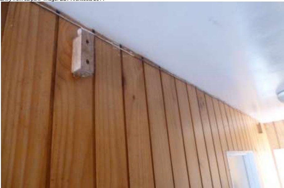
Laundry wall paneling + bracket, Image: B&T Architects 2014
