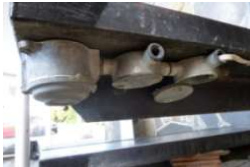
Stair landing (left) Garden irrigation system mounted under stair treads now defunct (right) Images: B&T 2014
