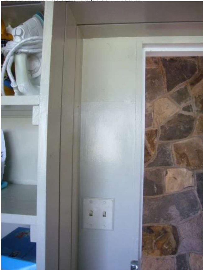
Door + view to stone wall in open lobby, Image: B&T Architects 2014
