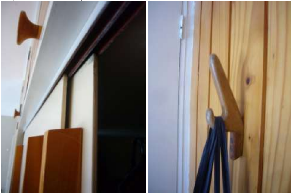
Wardrobe door detail showing turned wooden handles (left) Wooden coat hook (right) Image: B&T Architects 2014
