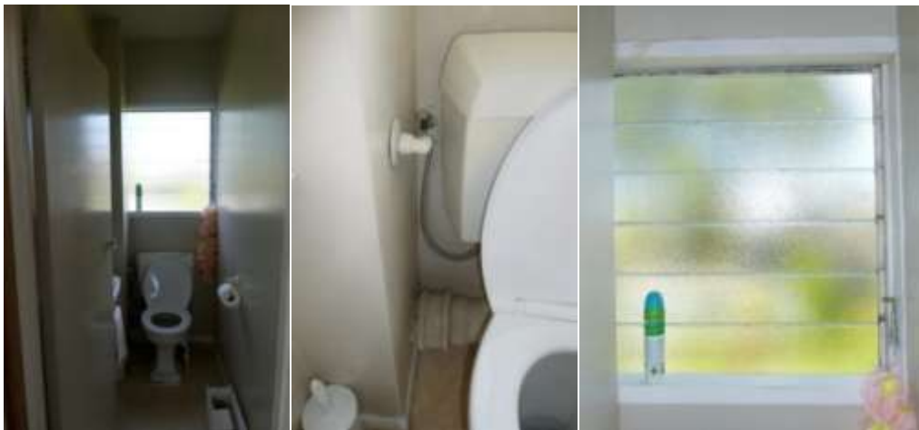
Toilet (left) Toilet connection (centre) Glass louver window (right) Images: B&T Architects 2014
