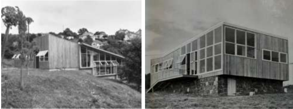
North façade of the Mrkusich House c.1950, Image: http://homenewzealand.blogspot.co.nz (left) Brenner's 'Paul house' Temple St (1950) Harold Paton photo, Image: www.lostproperty.org.nz
