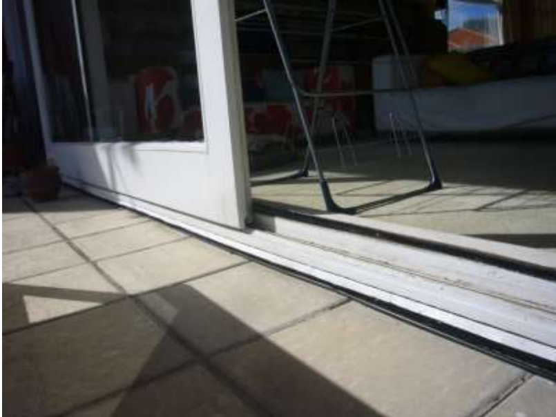
Sliding door opening, Image: B&T Architects 2014
