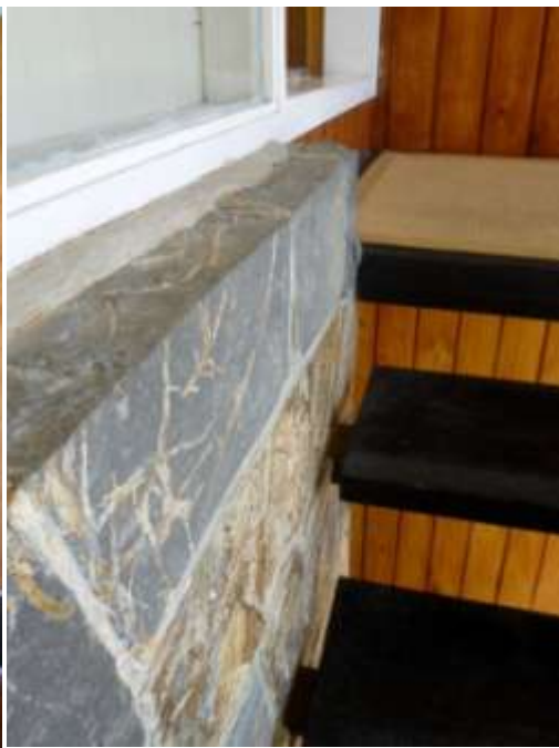
Showing stair and pipe hand rail (left) Stair tread connection to bluestone wall (right) Images: B&T 2014
