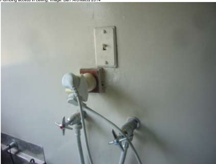
Bakelite power point mounted on wooden block, Image: B&T Architects 2014
