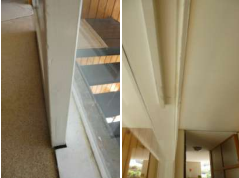
Sliding door open (left) Sliding door guide moulding (right), Images: B&T Architects 2014
