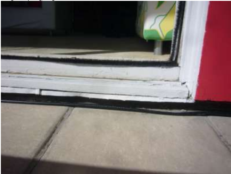
Sliding door threshold, Image: B&T Architects 2014
