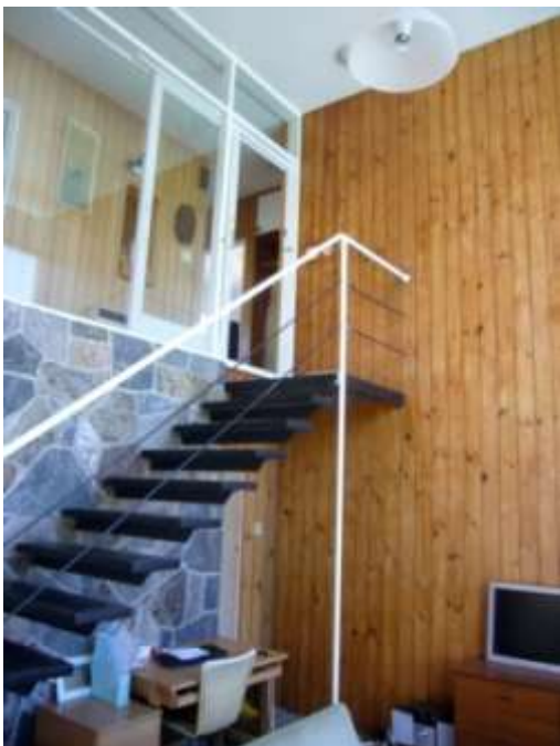
Showing stair and pipe hand rail (left) Stair tread connection to bluestone wall (right) Images: B&T 2014
