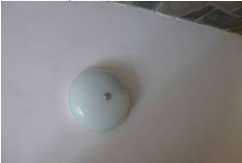
Light fitting fitted by Bob Simpson, east end of hall, Images: B&T Architects 2014
