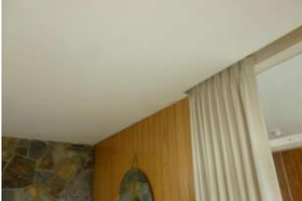
Ceiling at North West corner, Image: B&T Architects 2014
