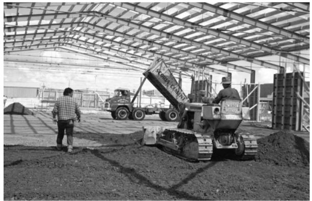
Additions to LynnMall, work in progress. Contractors at work concreting inside the new building for New Lynn's shopping mall, showing two workers, one of whom is operating a builldozer levelling out base course beneath the girder framework of the roof with a tip truck in the background. The contractors are Wilson Rothery Ltd. of Ellerslie. November 1969. Image: J. T. Diamond Collection JTD-11A-04016-1
