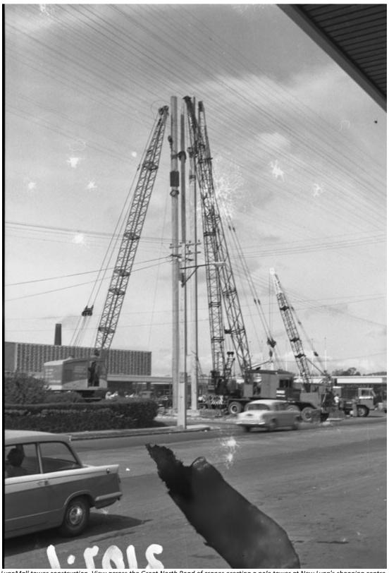
LynnMall tower construction. View across the Great North Road of cranes erecting a pole tower at New Lynn's shopping centre.
