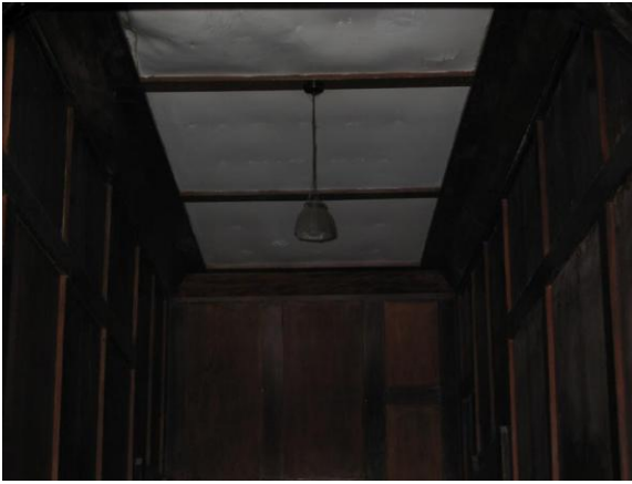
Warped ceiling panels in passageways, photos Graeme Burgess.
