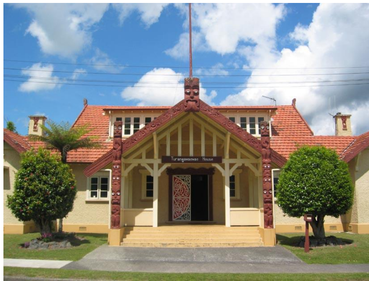
Entry porch. Photo: Graeme Burgess, 2006.
