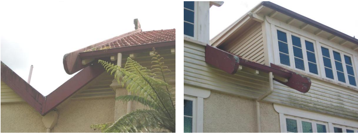
left: valley intersection with rainwater head behind, right: eaves between the clerestorey/dormers. Photos Graeme Burgess
