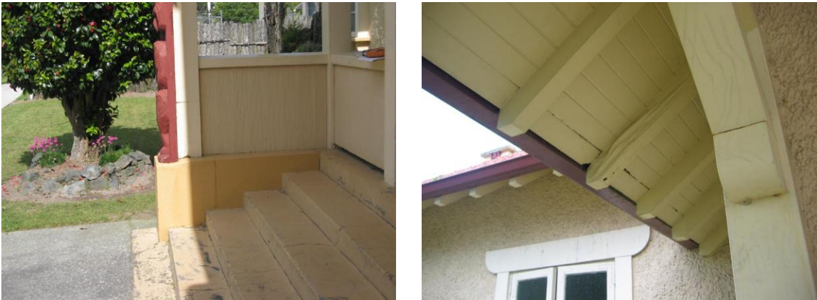
left: steps and side detail, note the post repair, right soffit detail, note decayed rafter photos Graeme Burgess.
