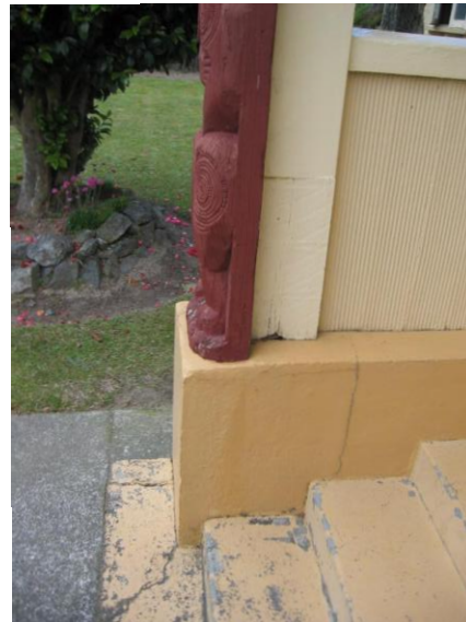
Left, Entry Porch rafters, right entry porch repaired post base, photos Graeme Burgess.
