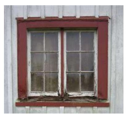
South window detail with rotted frame, sill and facings.
