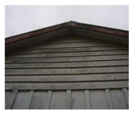
Weatherboards on southern gable end. Note the lack of flashings on butted boards Burgess & Treep, July 2012
