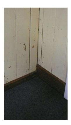
Corner detail showing uneven skirting, and split boards Burgess & Treep, July 2012
