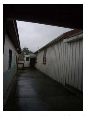
Concrete path on eastern side between the Wharenui and the wharepaku looking south, note concrete has been built up against the cladding
